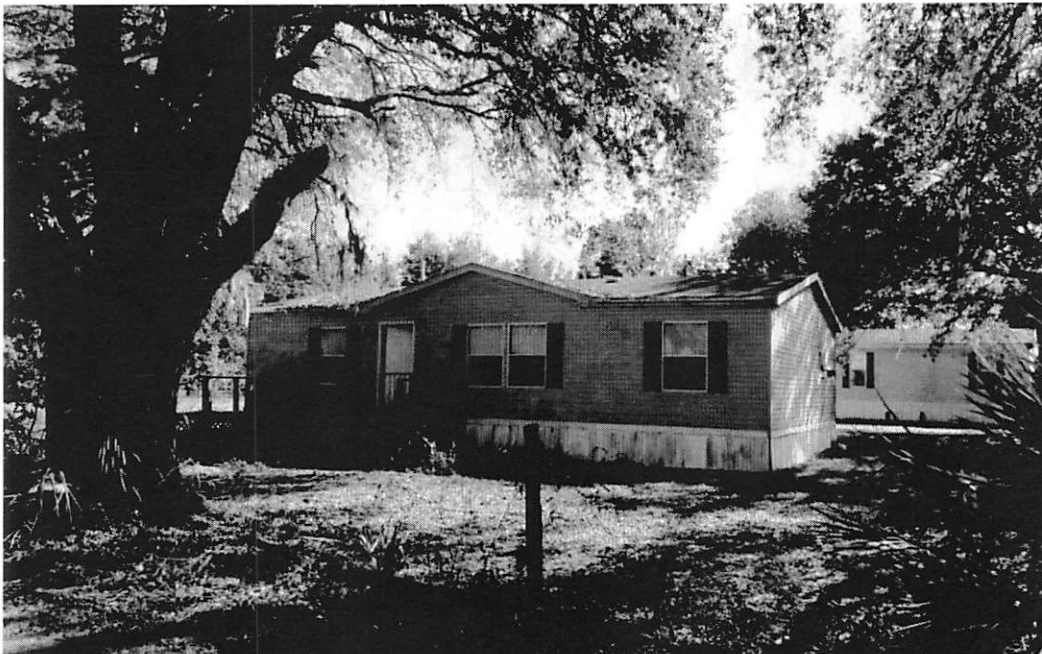
One of several mobile homes on property to the South of Subject Property (911 Halsema Road)
